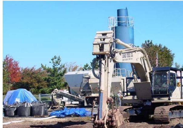
SSTT provided stabilization recipe design, pilot testing, field supervisor and reagent procurement for the in-situ treatment and processing of arsenic- and lead-bearing soil at the Weymouth Neck Project. The stabilized soils were tested by both TCLP and SPLP methods, and the treated soil passed MA GW-3 groundwater standards and RCRA TCLP levels for on-site reuse. Treatment operations were performed in-situ to depths of 15' with specialized slurry/mixing equipment.
